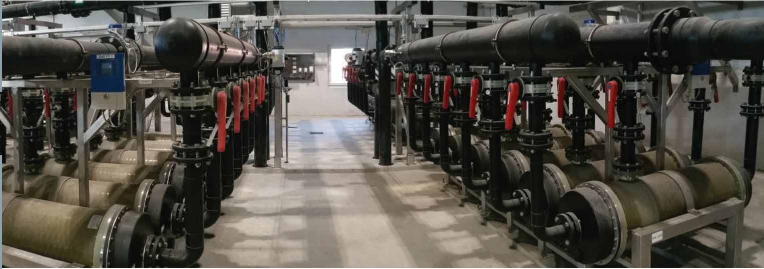
Metal transformation plant SWEDEN
